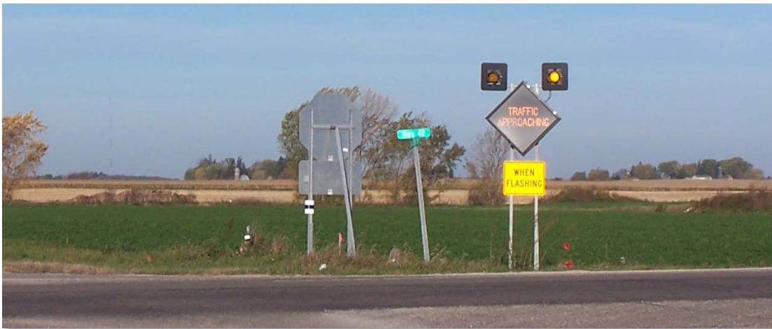
Figure 15: Rural intersection conflict warning system (RICWS) sign
