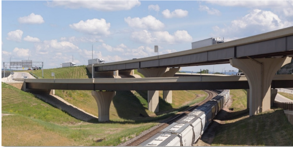
Figure 11: Highway interchange in Dresbach
